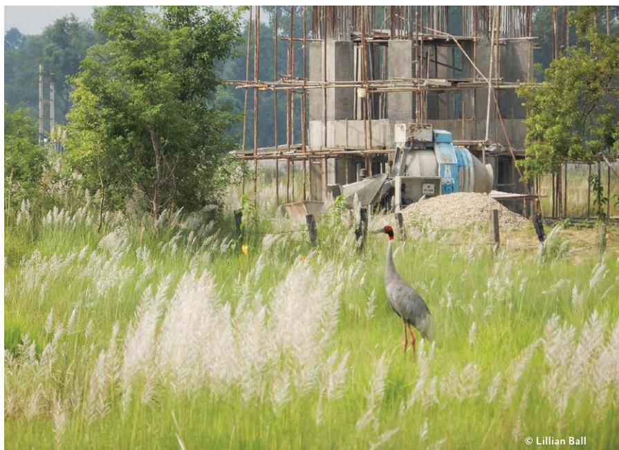
Construction underway in the Lumbini Sarus crane habitat
